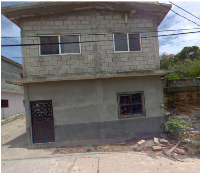
(a) A Confined URM building
